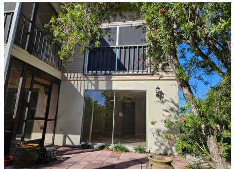
No Protection Throughout
