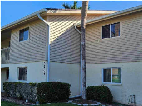
No Protection Throughout
