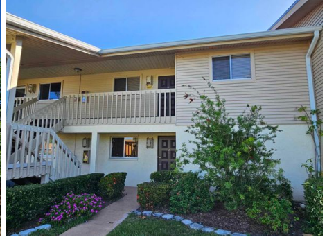
No Protection Throughout
