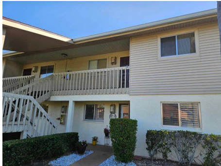
No Protection Throughout
