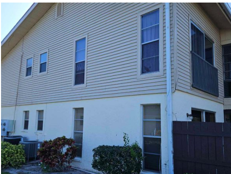
No Protection Throughout
