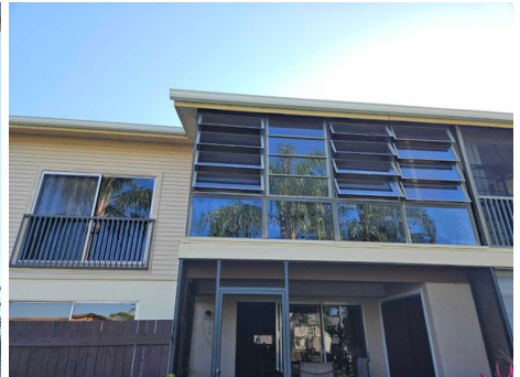
No Protection Throughout
