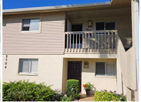
No Protection Throughout
