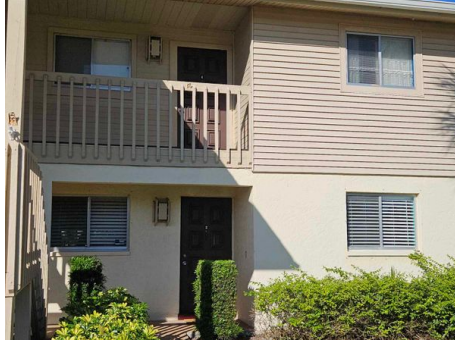
No Protection Throughout
