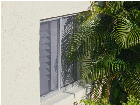
No Protection Throughout
