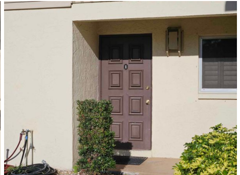
No Protection Throughout
