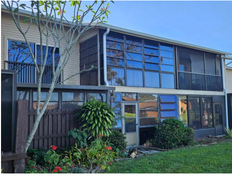
No Protection Throughout
