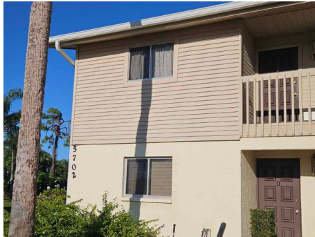
No Protection Throughout
