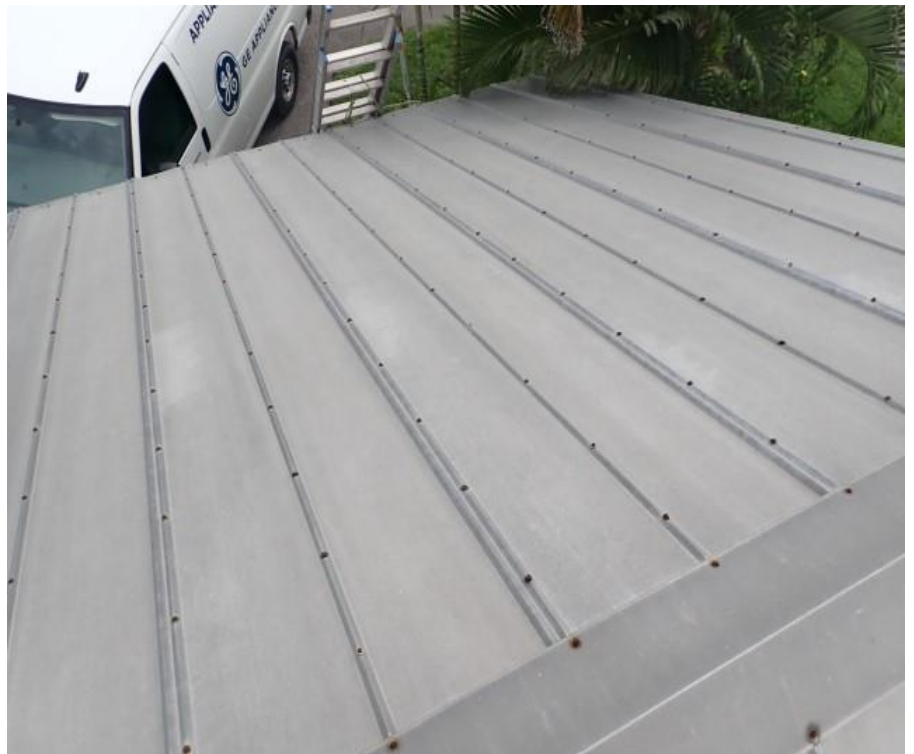
12. Bldg 4 - Garage C roof system overview
