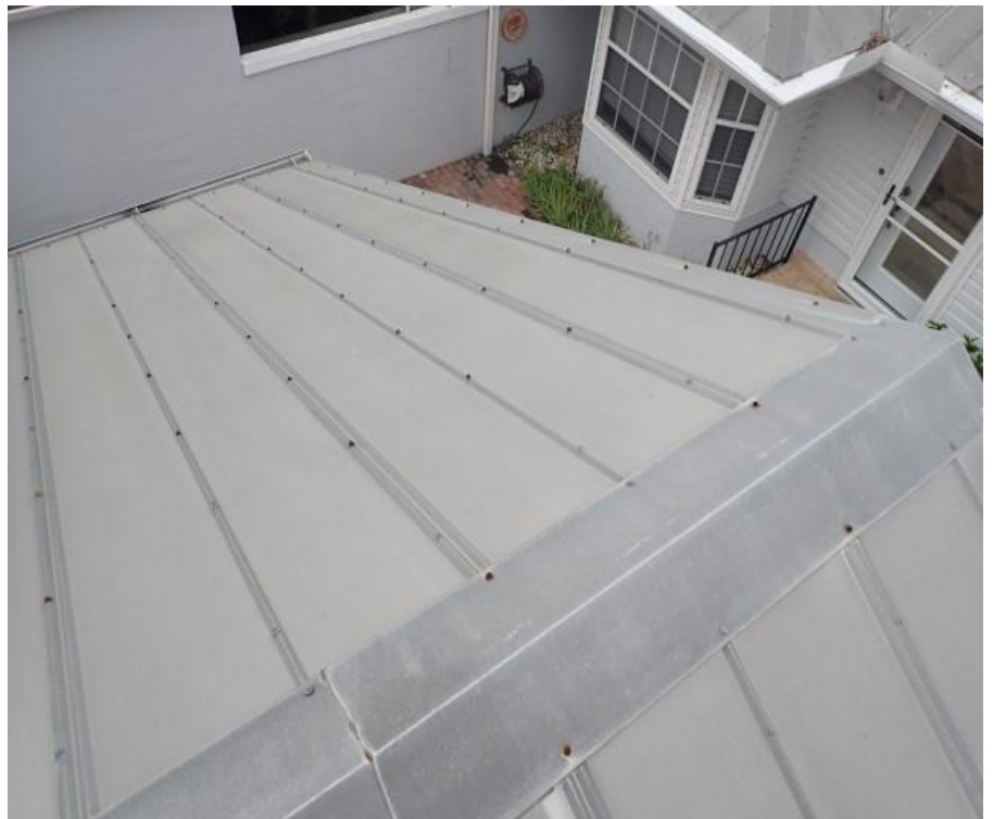
8. Bldg 6 - Garage B roof system overview
