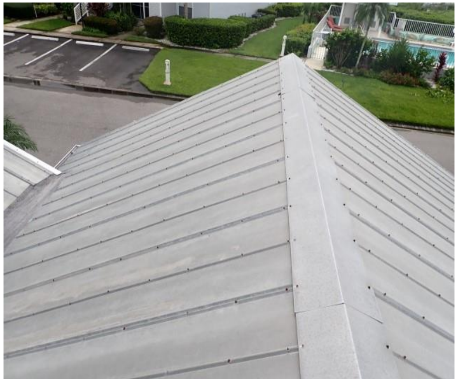
6. Bldg 5 - Garage B roof system overview
