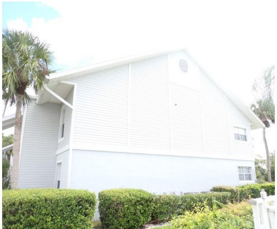
4. Building exterior side elevation overview
