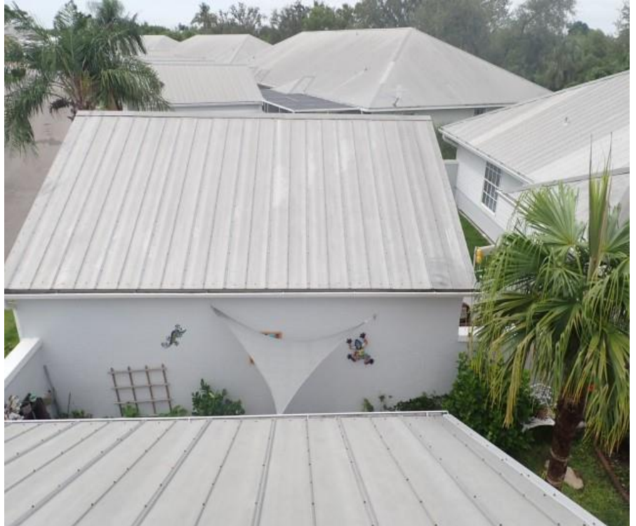
5. Bldg 5 - Garage A roof system overview
