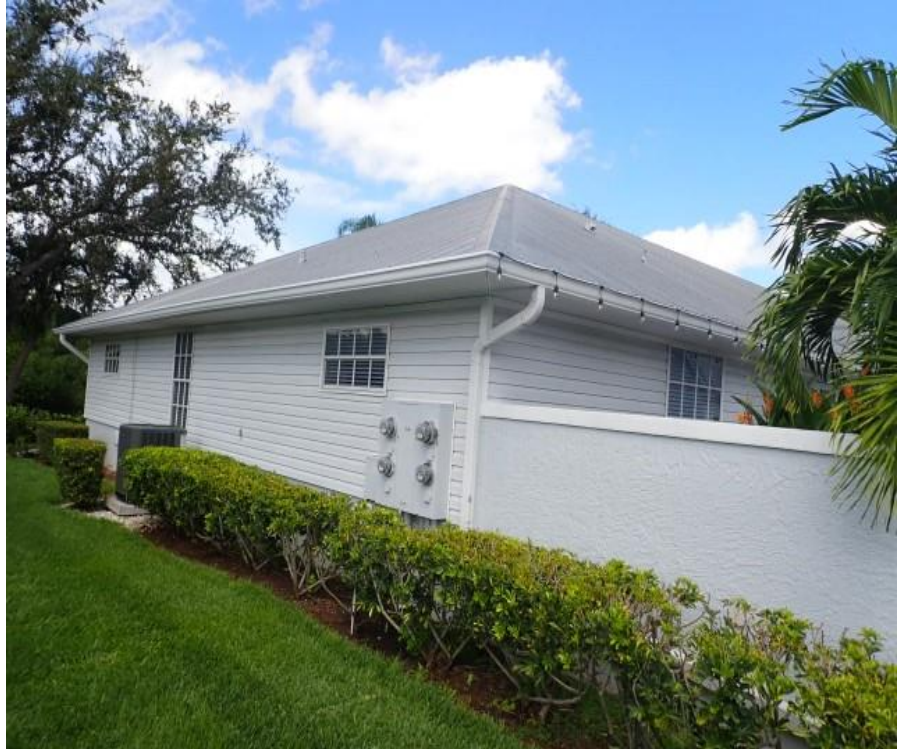
5. Building exterior side elevation overview
