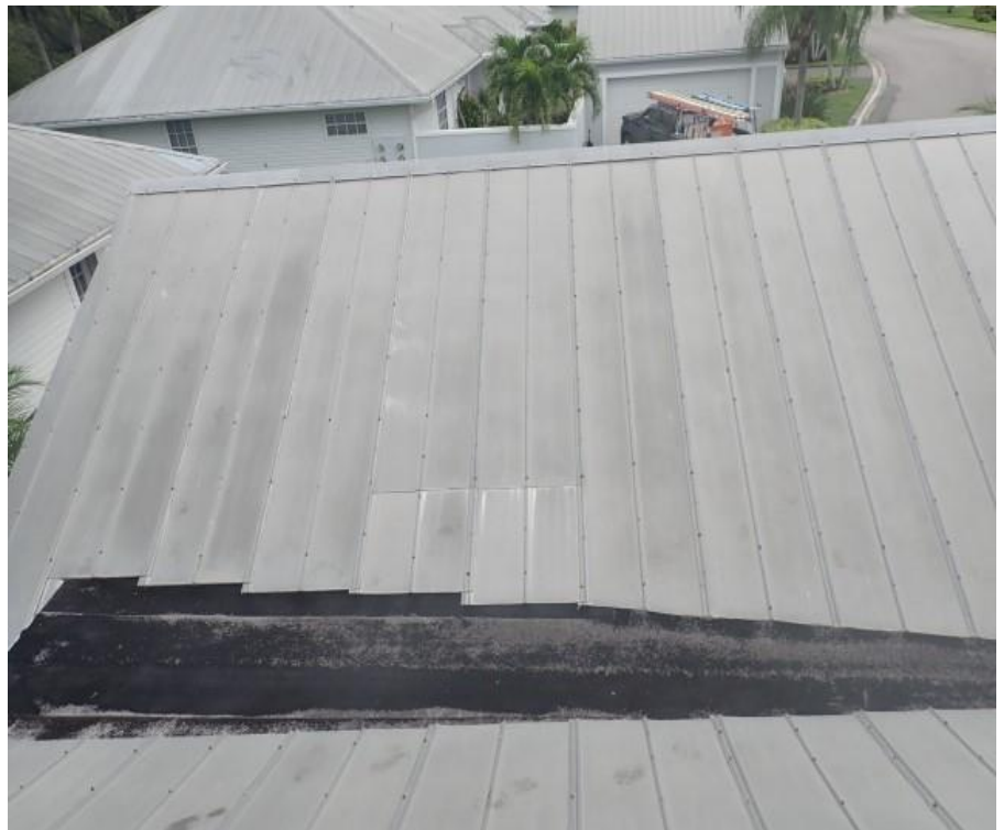
12. Bldg 10 roof system overview
