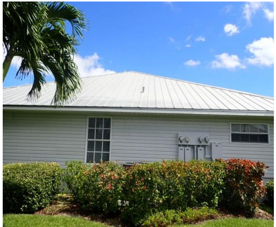
2. Building exterior side elevation overview
