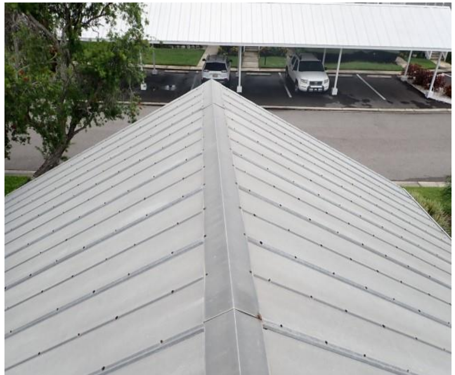
8. Bldg 4 - Garage B roof system overview
