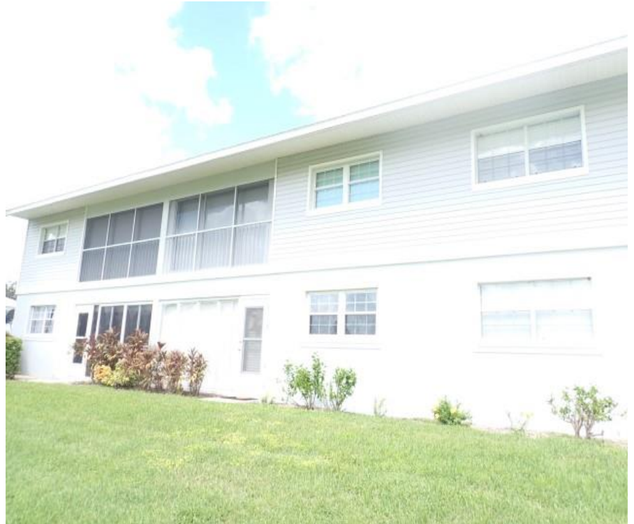
3. Building exterior rear elevation overview
