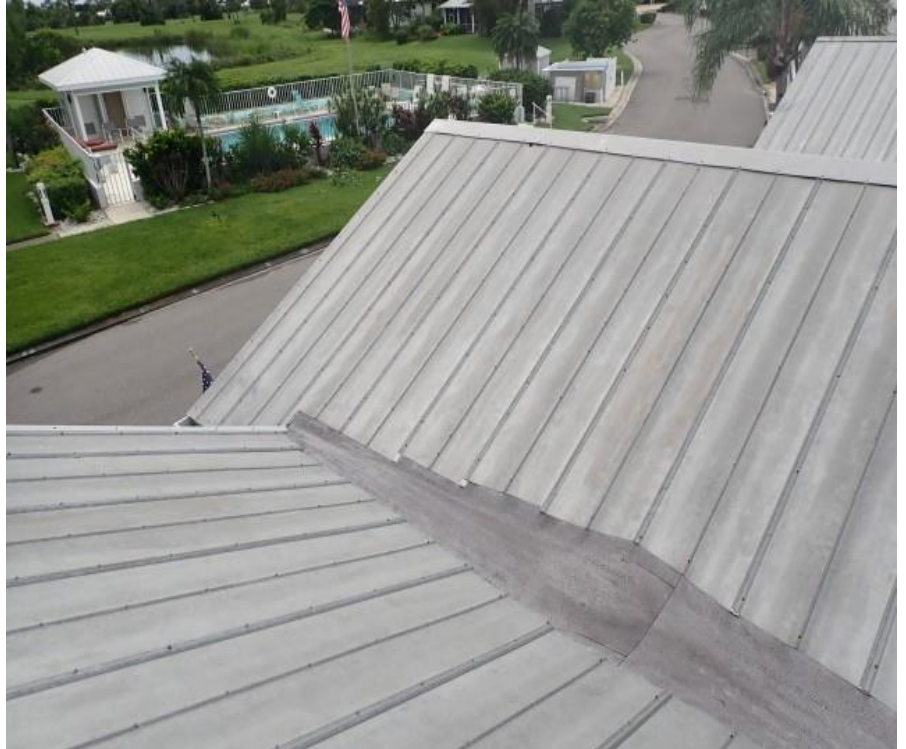
7. Bldg 5 - Garage B roof system overview
