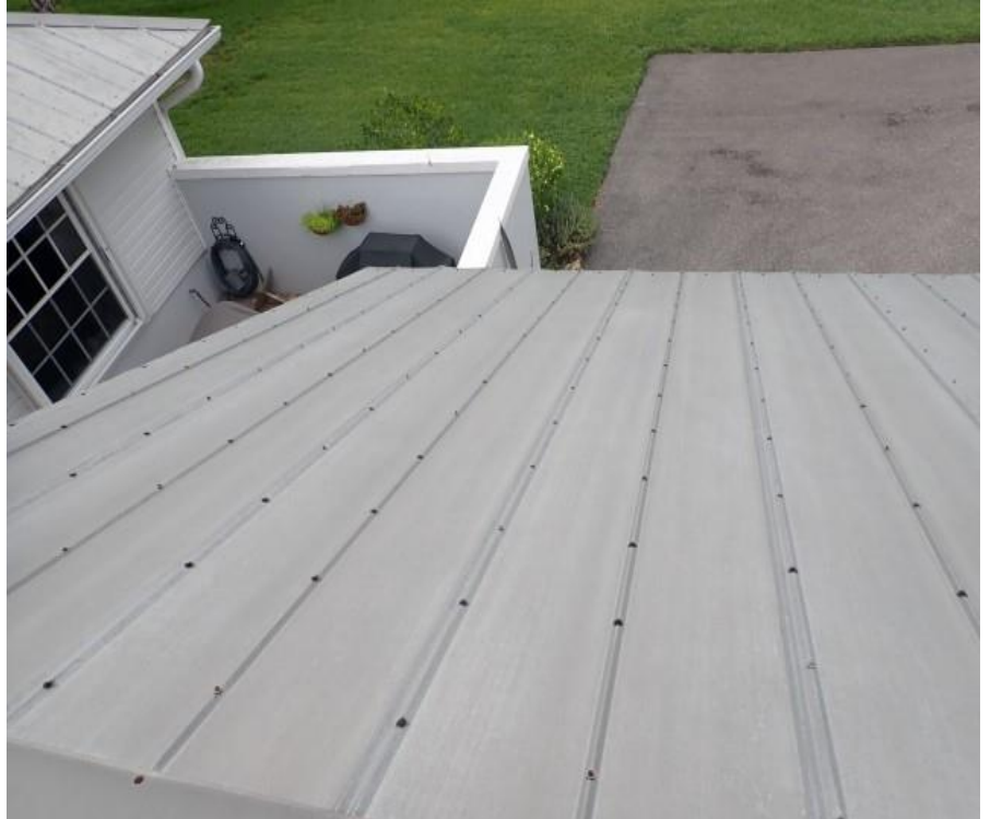
11. Bldg 2 - Garage C roof system overview
