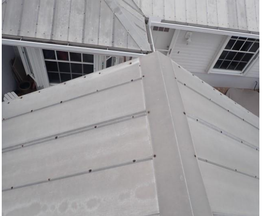
9. Bldg 2 - Garage B roof system overview
