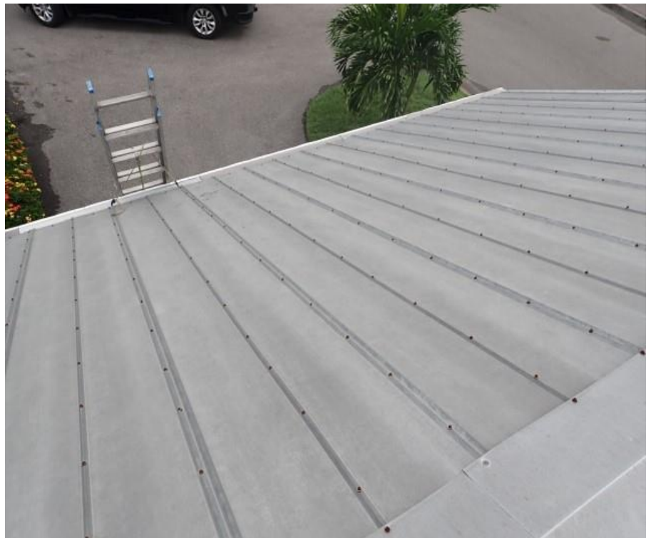
10. Bldg 5 - Garage C roof system overview
