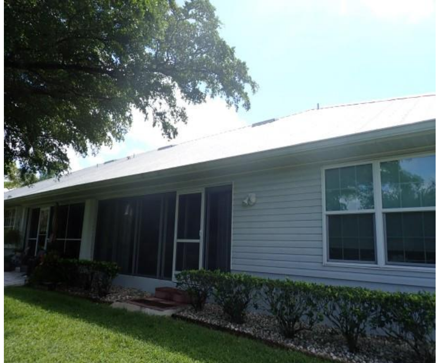
3. Building exterior rear elevation overview
