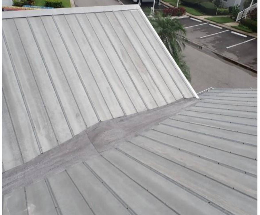
9. Bldg 5 - Garage C roof system overview
