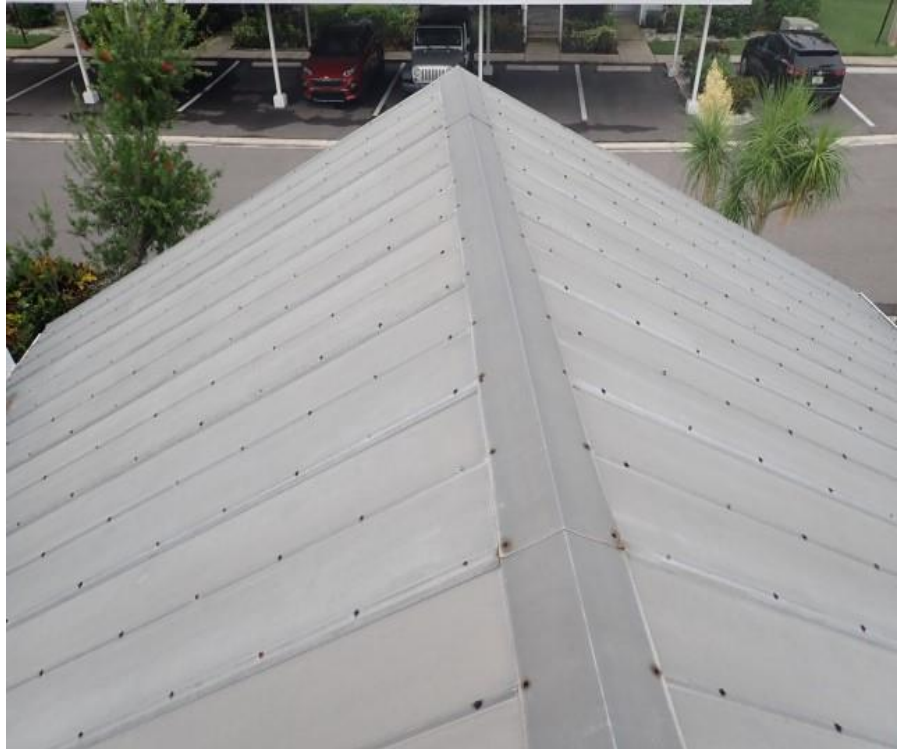
7. Bldg 2 - Garage B roof system overview
