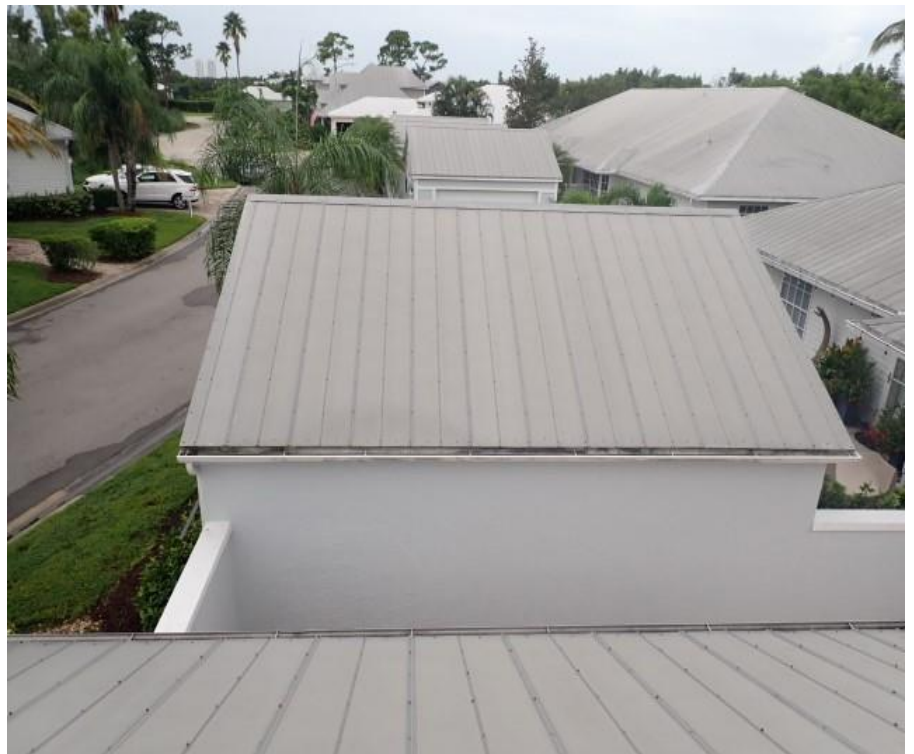
6. Bldg 8 - Garage A roof system overview
