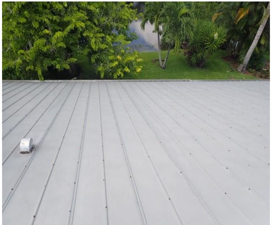
10. Bldg 10 roof system overview
