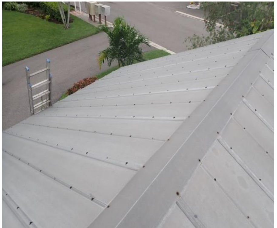
10. Bldg 2 - Garage C roof system overview
