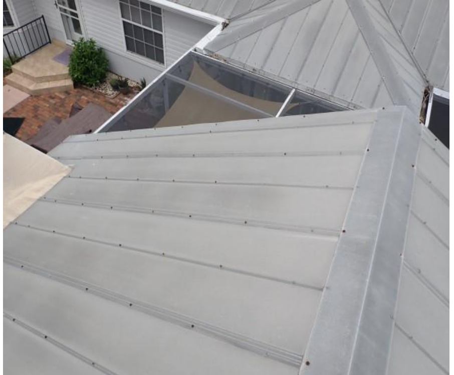
11. Bldg 6 - Garage C roof system overview
