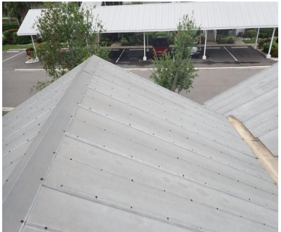
12. Bldg 2 - Garage C roof system overview
