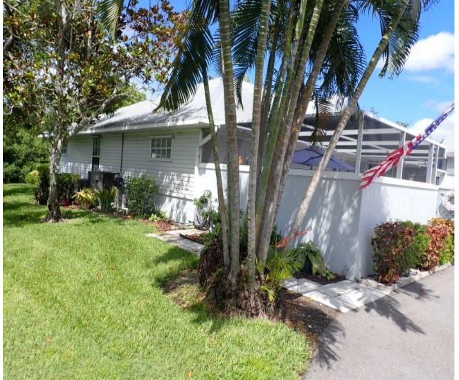
3. Building exterior side elevation overview
