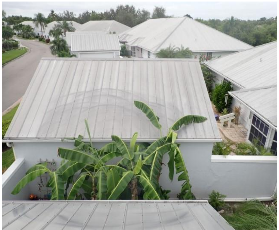
6. Bldg 4 - Garage A roof system overview
