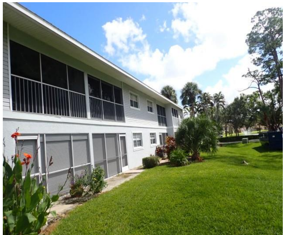
4. Building exterior rear elevation overview
