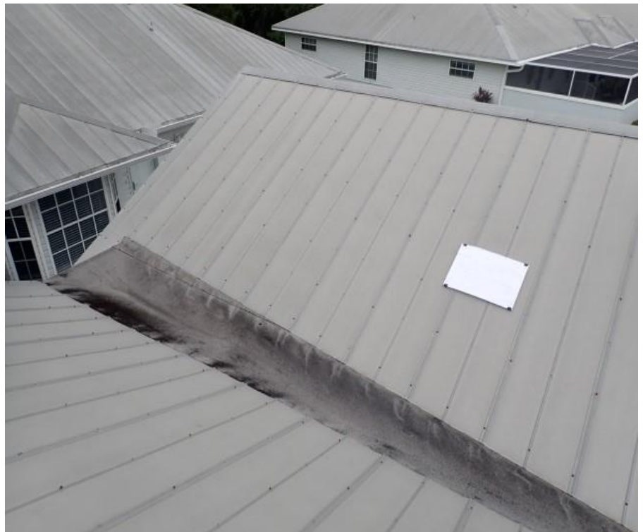
10. Bldg 8 - Garage C roof system overview
