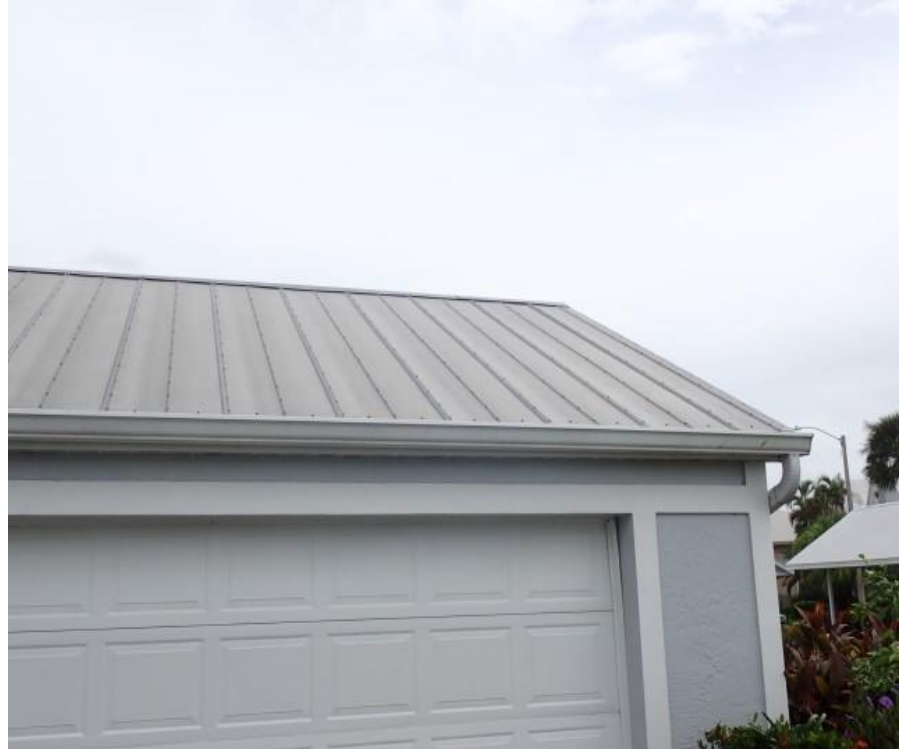
7. Bldg 4 - Garage A roof system overview
