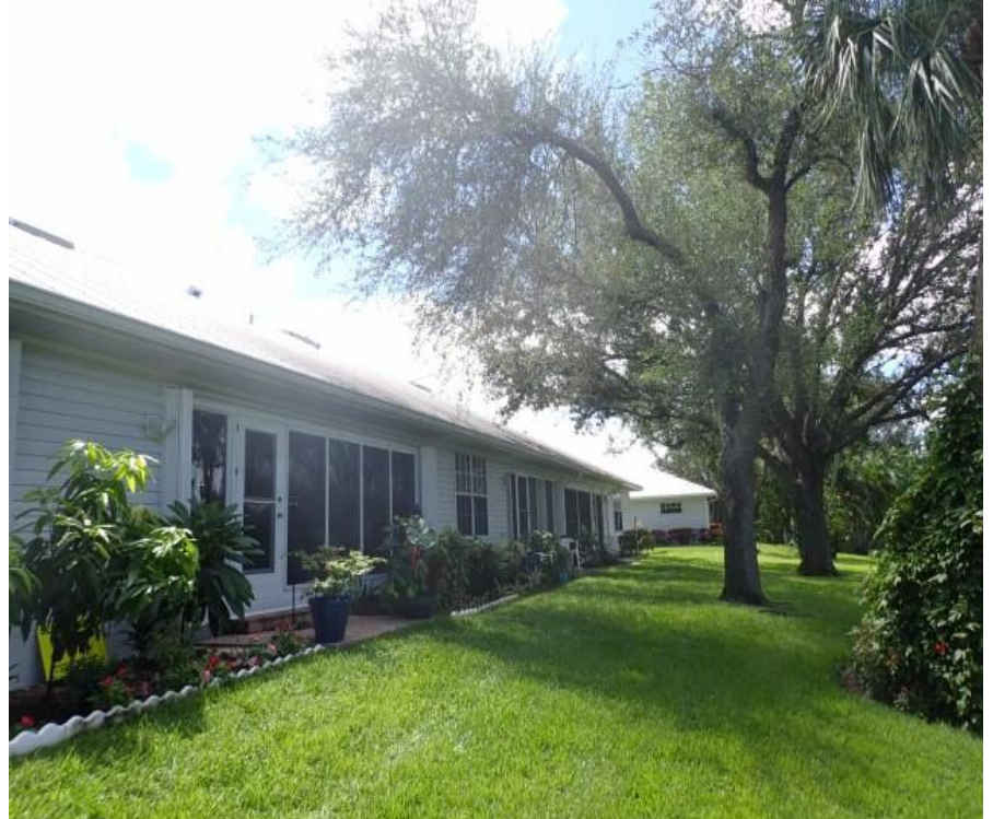
3. Building exterior rear elevation overview
