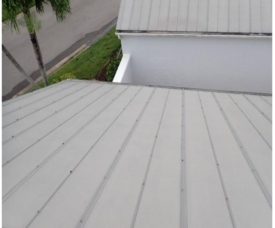
9. Bldg 8 - Garage B roof system overview
