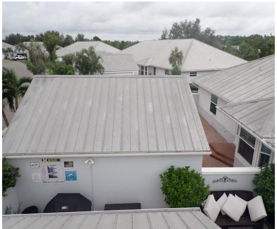
6. Bldg 2 - Garage A roof system overview
