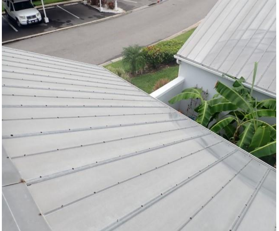
9. Bldg 4 - Garage B roof system overview
