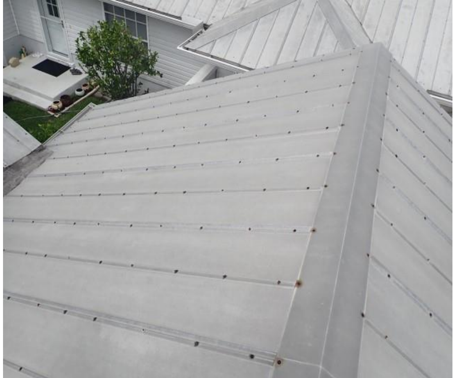
13. Bldg 4 - Garage C roof system overview
