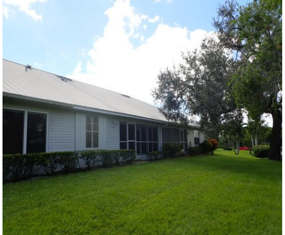
3. Building exterior rear elevation overview
