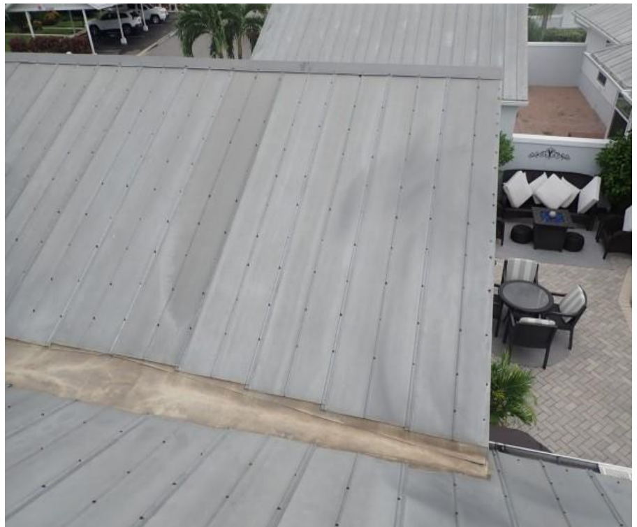
8. Bldg 2 - Garage B roof system overview
