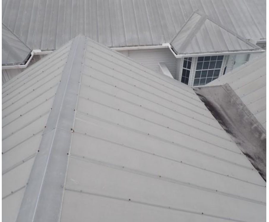
7. Bldg 8 - Garage B roof system overview
