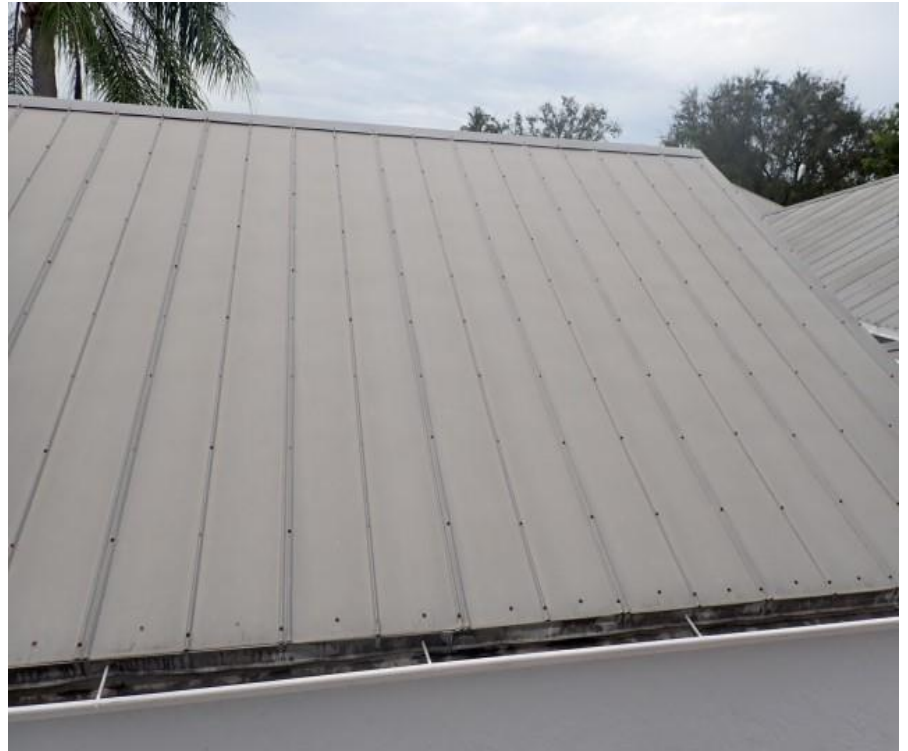
5. Bldg 6 - Garage A roof system overview
