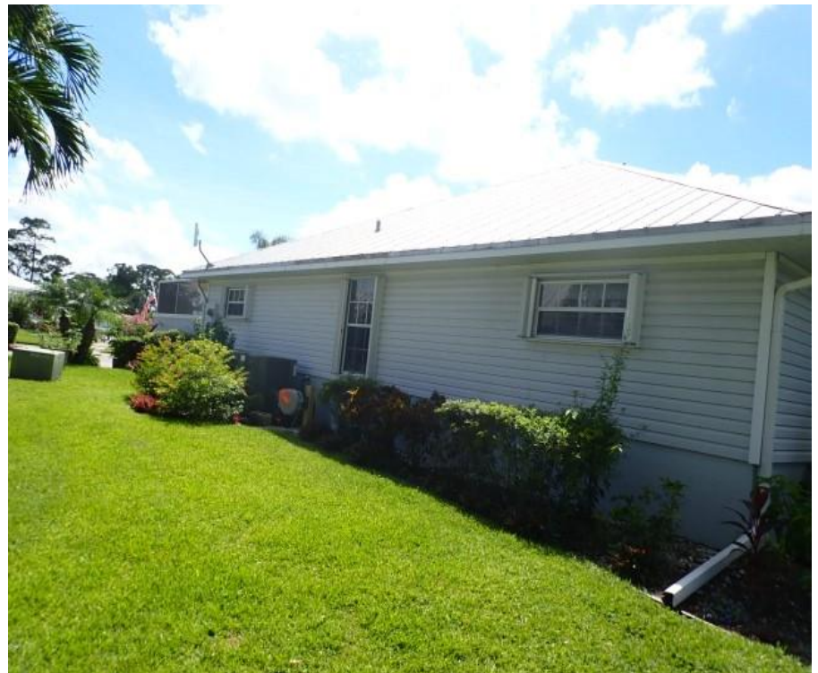
4. Building exterior side elevation overview
