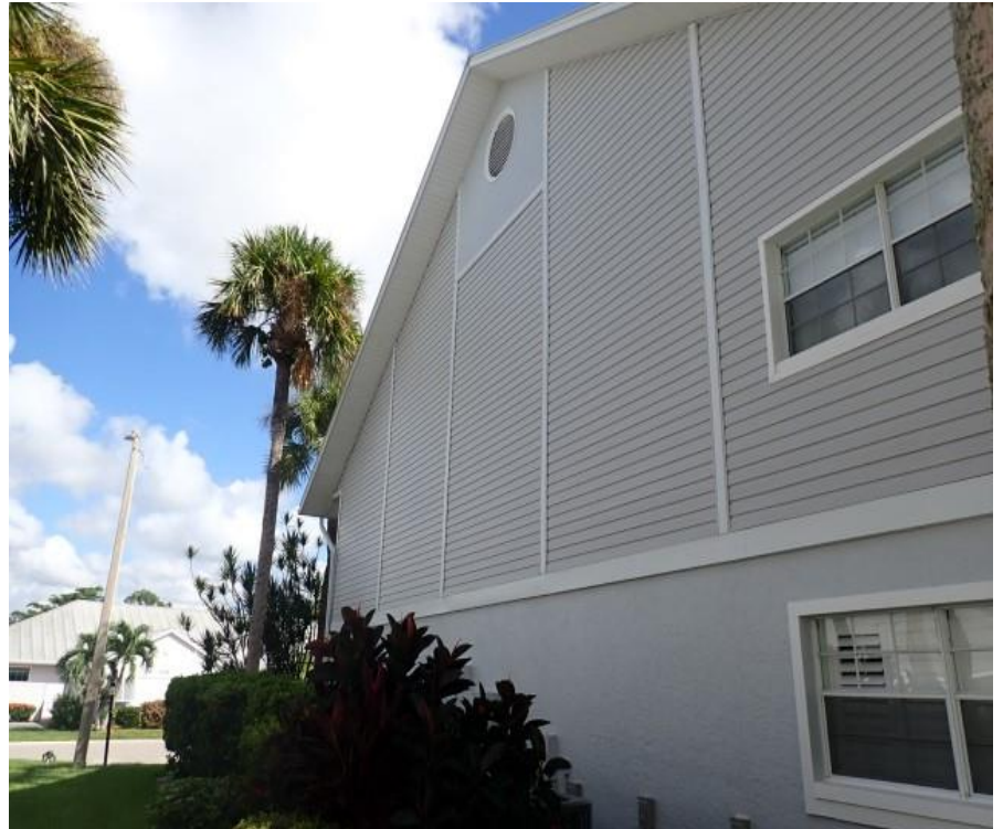
5. Building exterior side elevation overview
