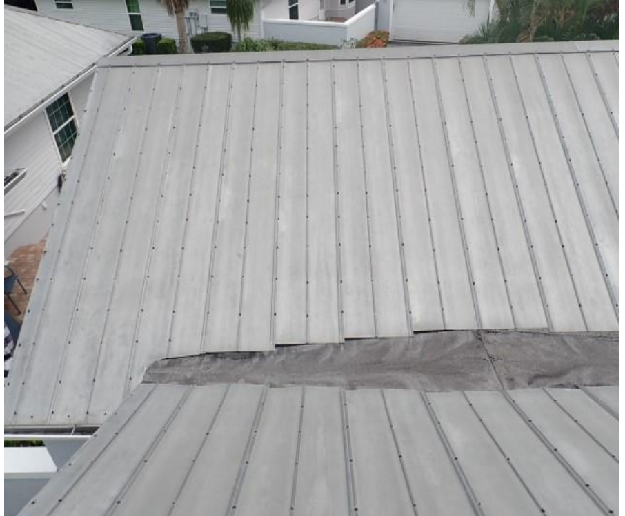
11. Bldg 4 - Garage C roof system overview
