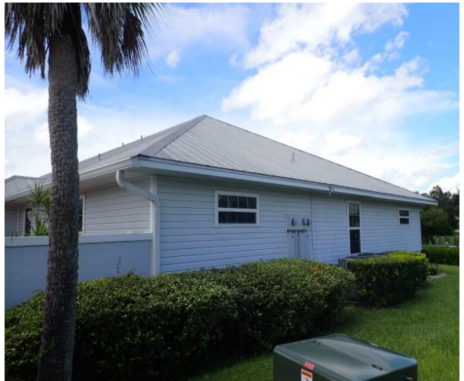
4. Building exterior side elevation overview
