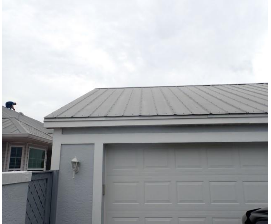
5. Bldg 2 - Garage A roof system overview
