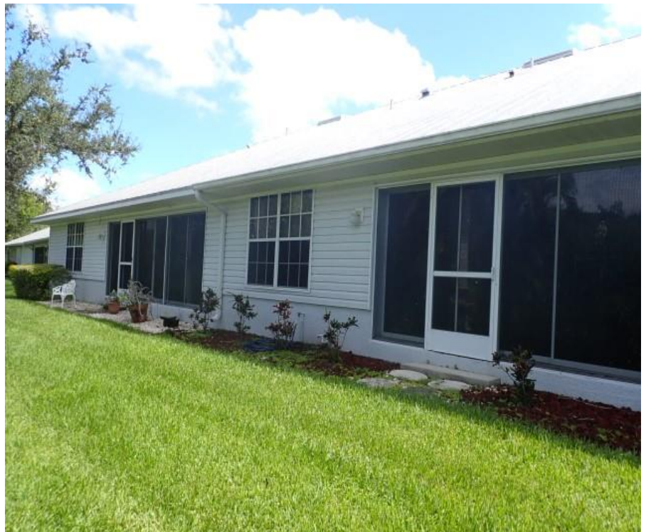
4. Building exterior rear elevation overview
