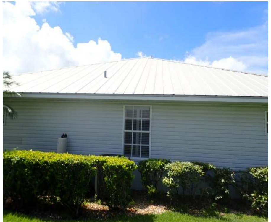
4. Building exterior side elevation overview
