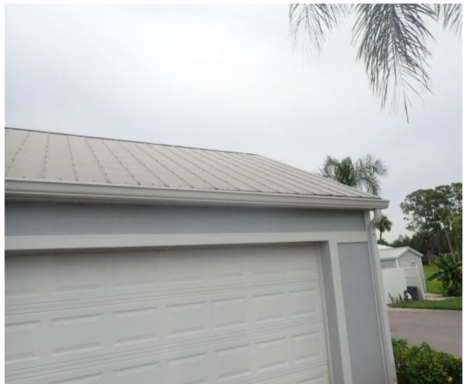
6. Bldg 6 - Garage A roof system overview
