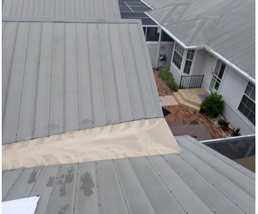
9. Bldg 6 - Garage B roof system overview
