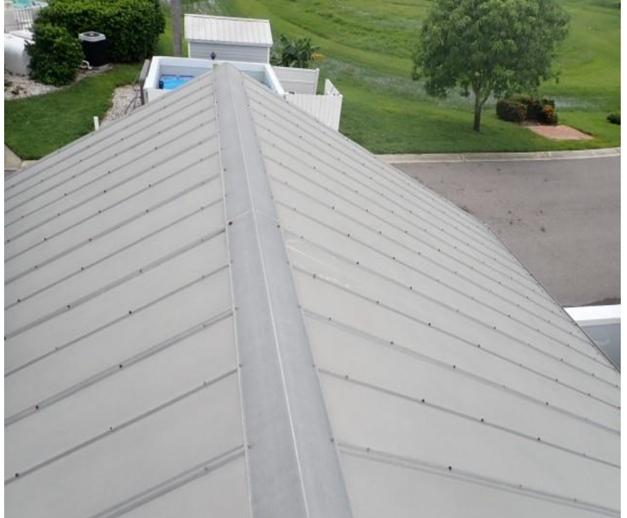
7. Bldg 6 - Garage B roof system overview
