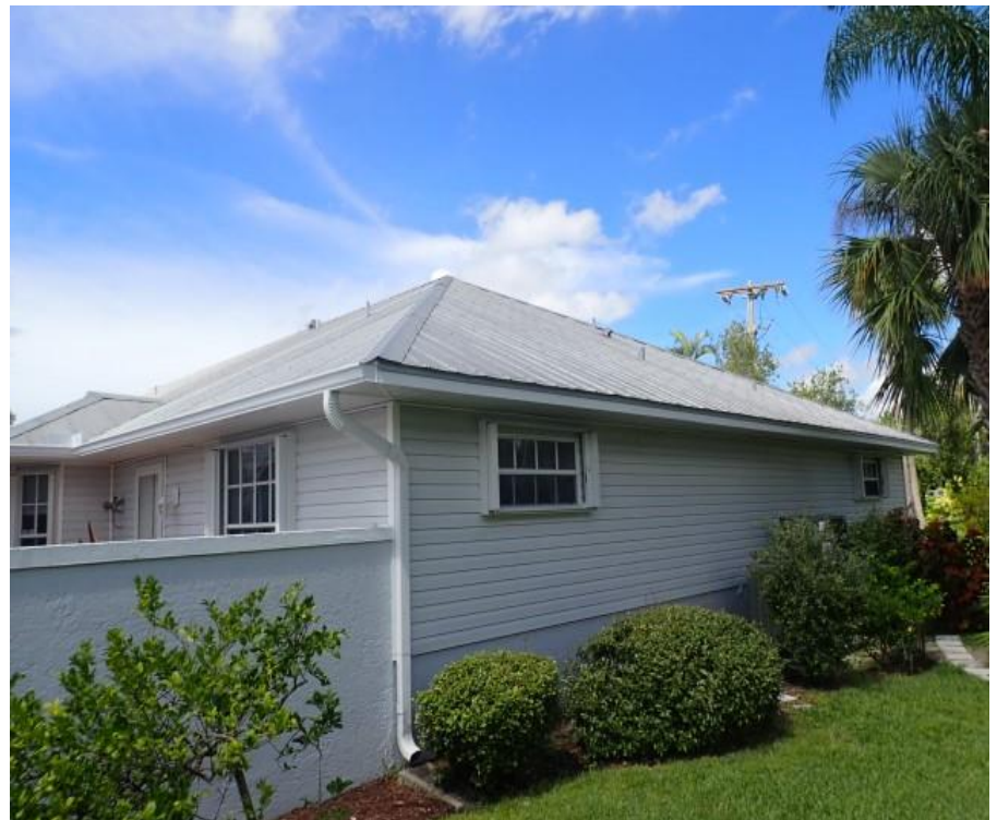
4. Building exterior side elevation overview
