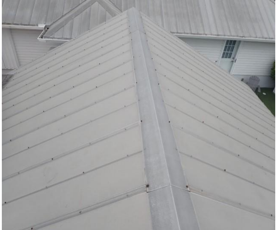
11. Bldg 8 - Garage C roof system overview
