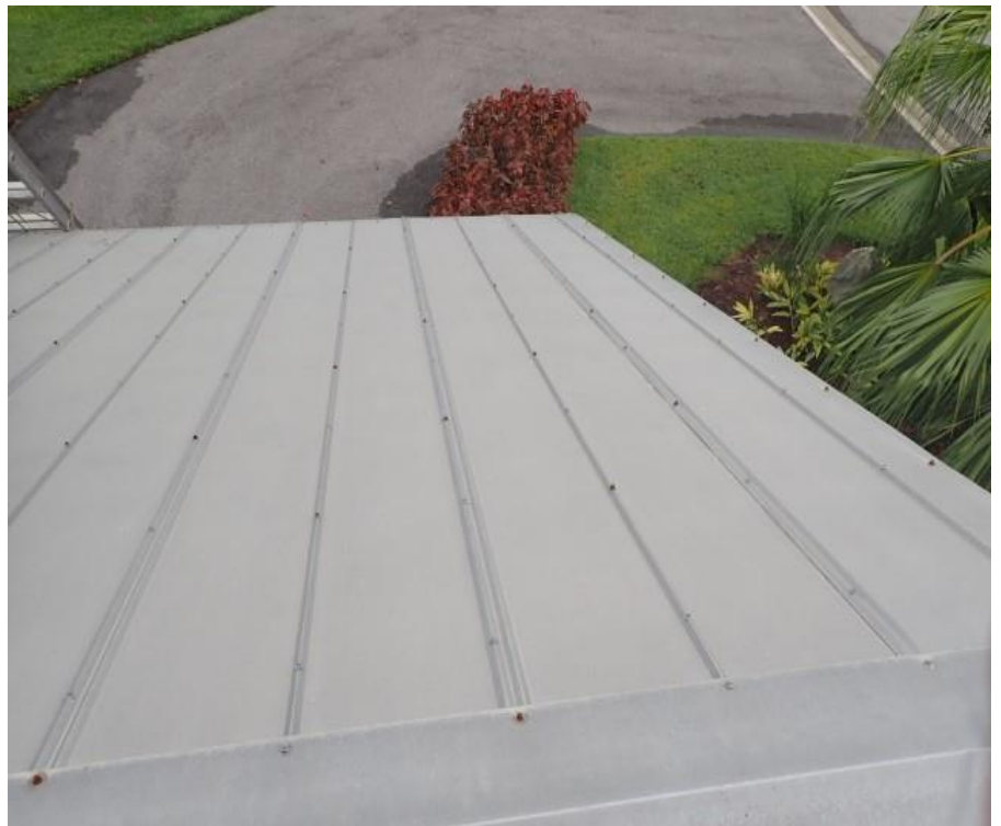
12. Bldg 8 - Garage C roof system overview
