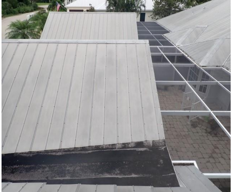
11. Bldg 10 roof system overview
