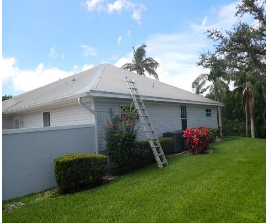
5. Building exterior side elevation overview
