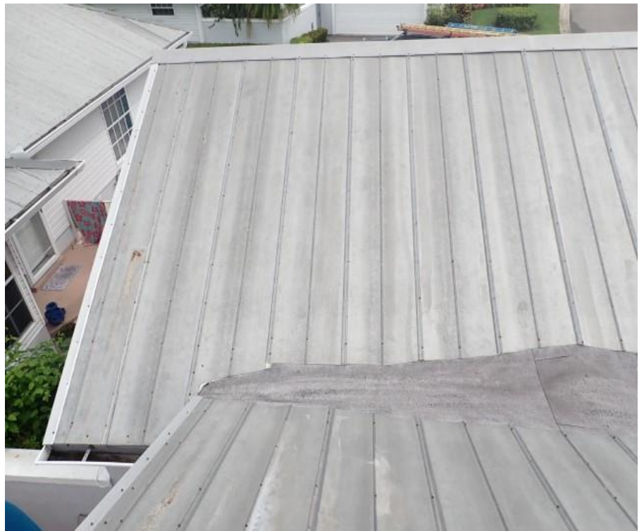
8. Bldg 5 - Garage C roof system overview
