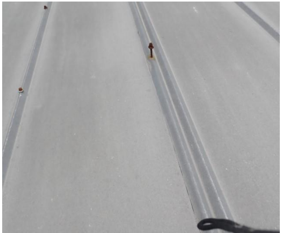
18. Deficiency #1 - Loose fasteners
