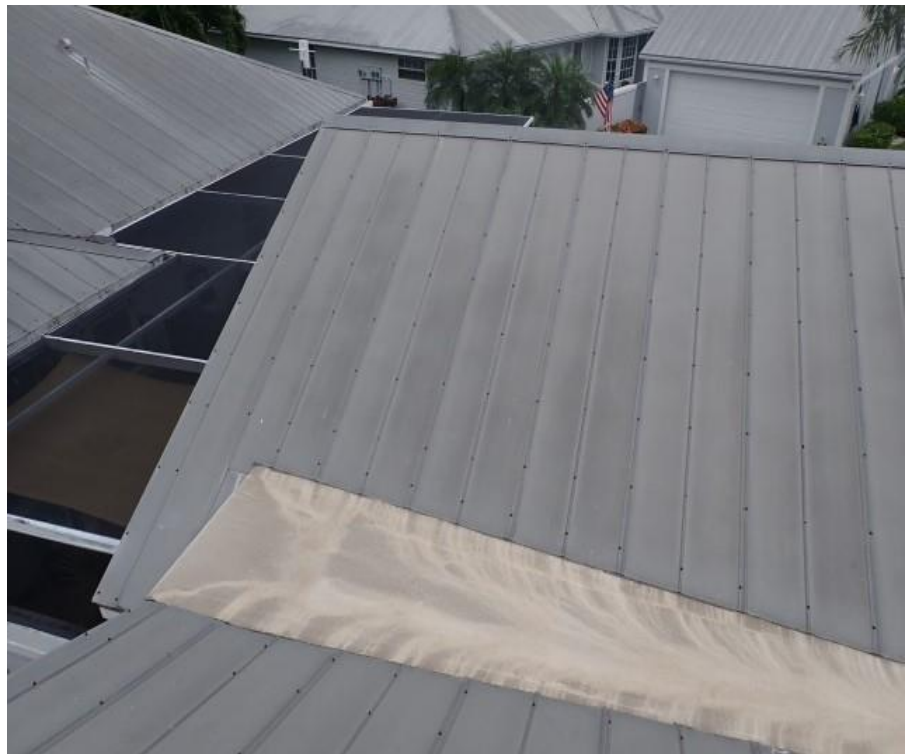
10. Bldg 6 - Garage C roof system overview
