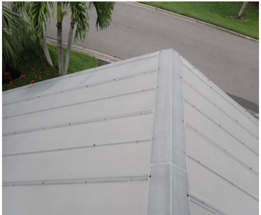
8. Bldg 8 - Garage B roof system overview
