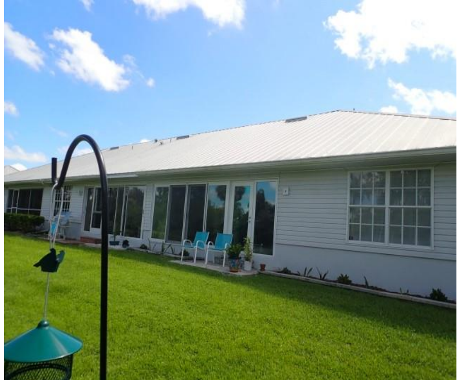
3. Building exterior rear elevation overview
