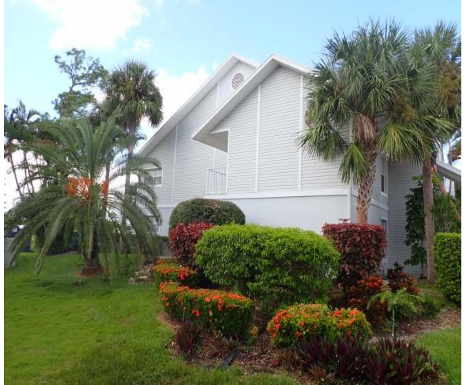
3. Building exterior side elevation overview
