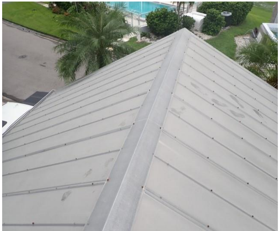
12. Bldg 6 - Garage C roof system overview
