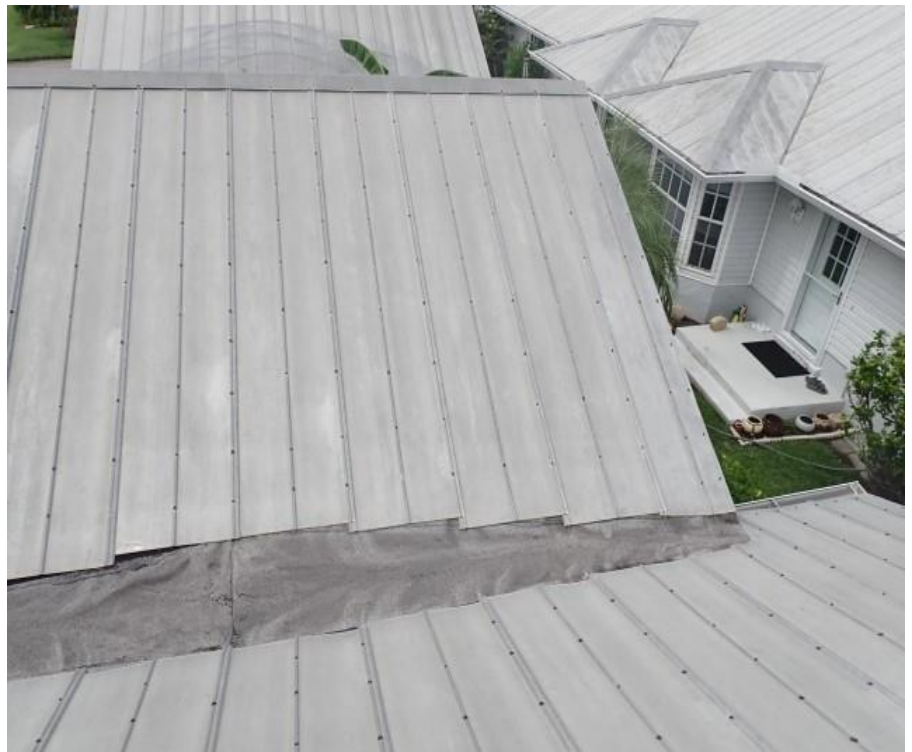
10. Bldg 4 - Garage B roof system overview
